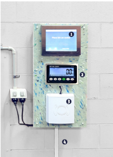
The weighing indicator, RFID scanner and the touchscreen PC are housed with the mounting plate which is mounted to the wall with 6 screw points (hardware dependent on wall - installation specifics to be confirmed at preliminary site visit)
